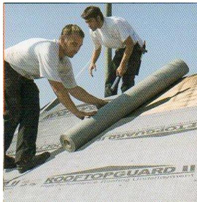
**SITE PROTECTION:** Prior to loading the roofing materials onto the RoofTopGuard product, it is recommended that a roof jack, with planks, toe boards, or a strong platform be secured to the underlying roofing deck to prevent slippage of stored materials on steep sloped roofs (greater than 4 : 12 pitch). See OSHA regulations (Standard 29 CFR), fall protection systems criteria and practices – 1926.502.
